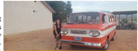
Cyndie breaking ground for a home for these two.
